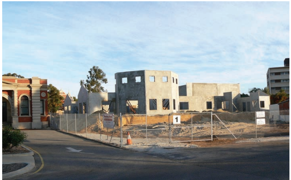
All the panels are in position in record time
