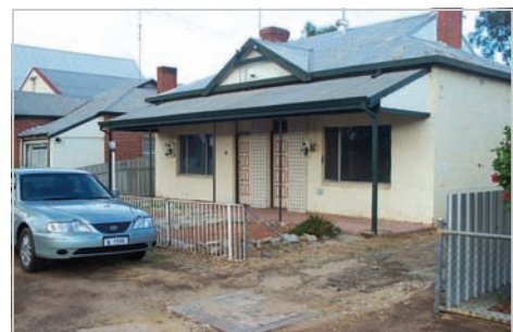
Demolition will start around 13th November
